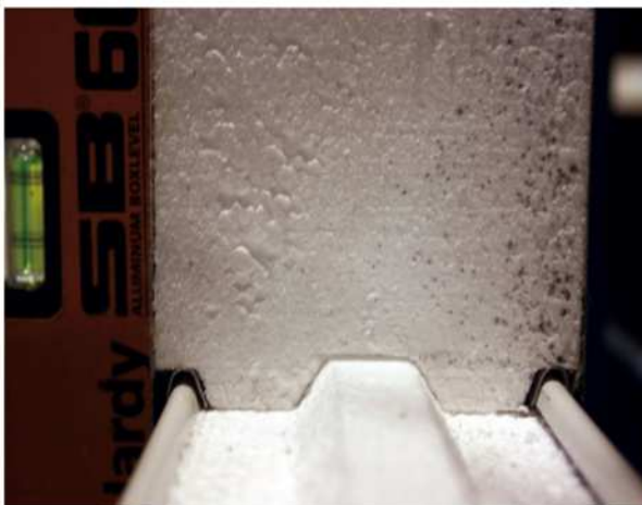
Thermo lock joint connection
