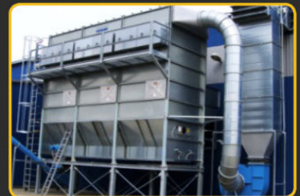
The veiw of the Dust collector (Bag filter type) 집진기(백필터 방식)
